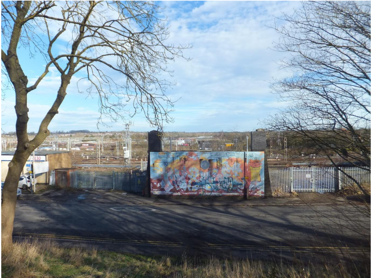
Figure 10 Looking at the gap across Abbey Street to the bridge support before the West Coast Main Line is reached by the GCR. Taken from the raised trackbed, at the northernmost walkable extent of this portion of the Great Central Walkway, looking north (SP 5161 7570).
