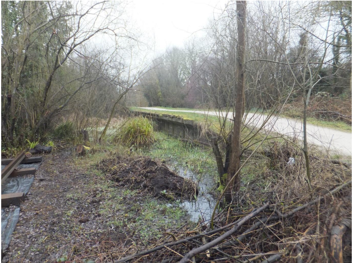
Figure 7 A closer look at the platform at the former Rugby Central station. Looking north from the trackbed (SP 5139 7447).
