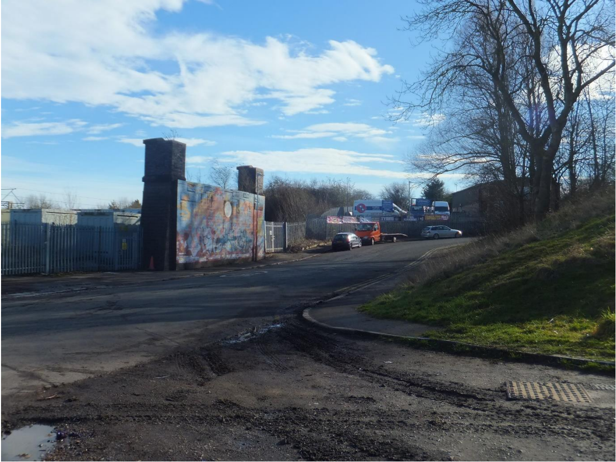
Figure 9 Remains of the bridge taking the GCR across Abbey Street just before it reaches the West Coast Main Line (SP 5161 7570).
