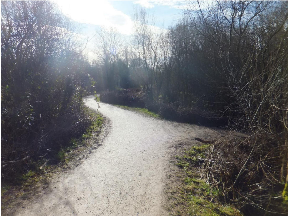
Figure 4 Looking south along the Great Central Walkway at the southernmost extent of the raised station platform. It shows how the walkway has been created to meander with vegetation and wetland in pockets on each side (SP 5139 7445).
