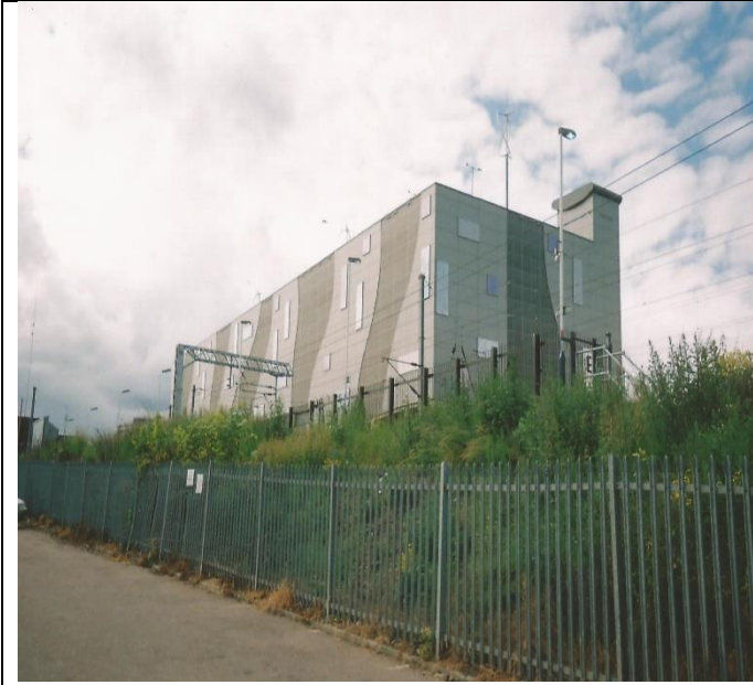
Caption Above: The stark 'box' of Luton's Car Park stack deals with security and capacity in one go as well as utilising limited land space. Like it or loathe it, it is functional. Luton is a growing population and needs better links.
