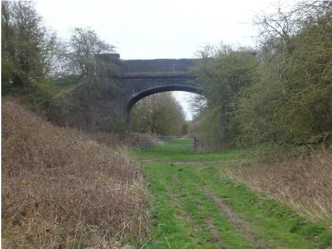
Figure 8 Looking south at the overbridge where the Jurassic Way crosses (SP 5429 5492).
