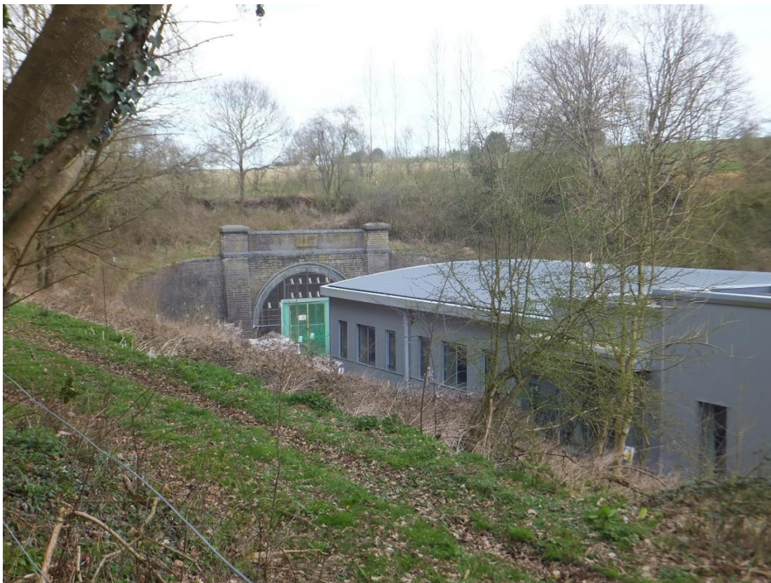
Figure 15 Looking east over the trackbed at the new building in front of the southern portal of Catesby Tunnel (camera at SP 5332 5690).
