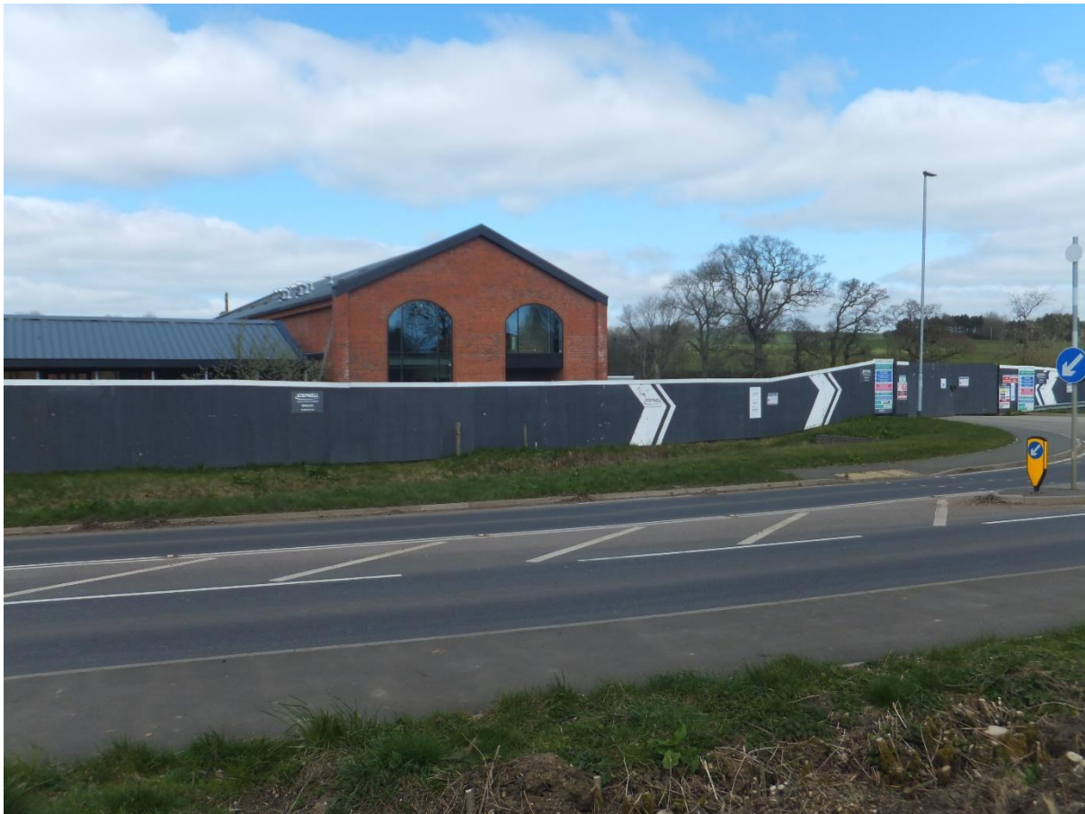
Figure 13 Looking north at the building at the front of the new development at Catesby Tunnel on the A361 near Charwelton (SP 5368 5612).
