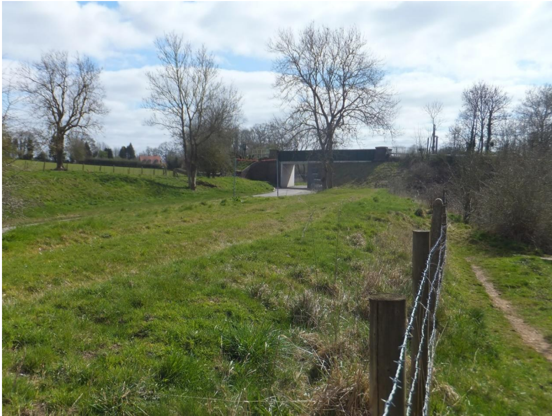
Figure 14 Looking south-east from the bridleway west of the railway cutting, showing the developed trackbed and the road bridge (camera at SP 5352 5640).
