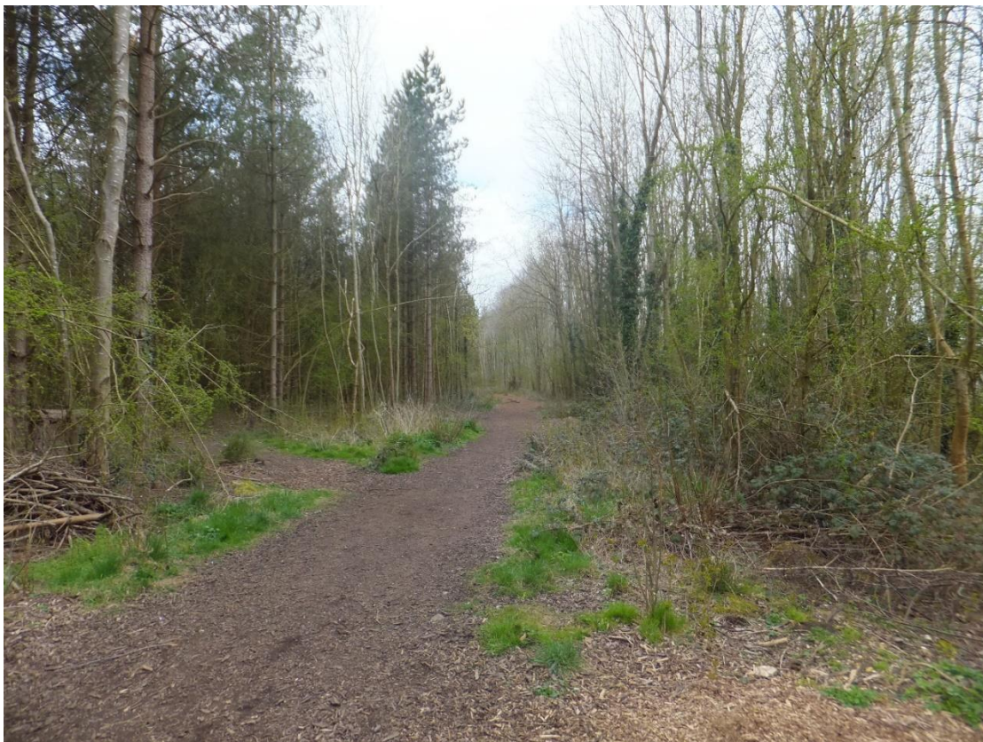
Figure 3 Looking north along the trackbed on the embankment in Woodford Halse (SP 5403 5263).
