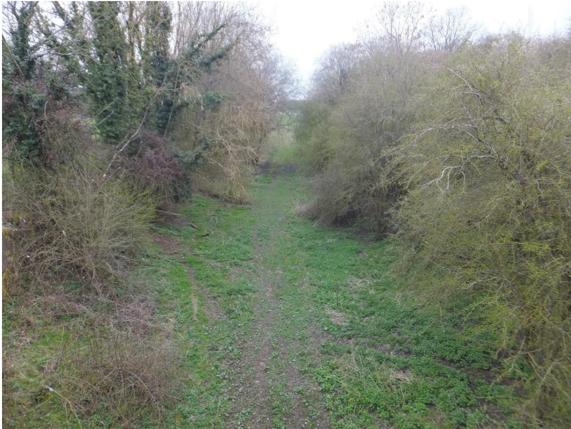
Figure 11 Looking north from the bridge over the trackbed on Church Street in Charwelton (SP 5384 5582).
