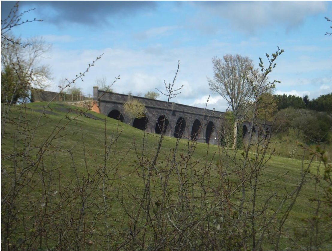
Figure 5 Looking north-west towards the southern end of Catesby Viaduct from close to the embankment (camera at SP 5225 6036).
