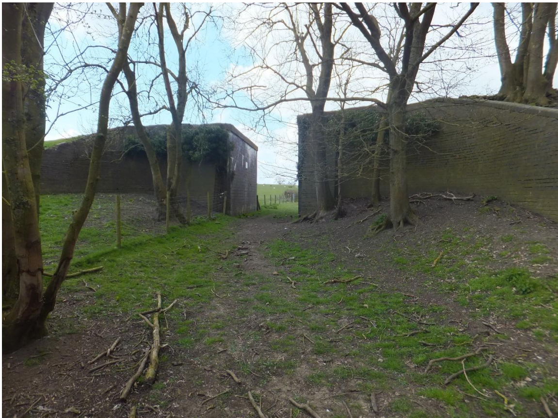
Figure 4 View west where the Jurassic Way passes through the GCR embankment (SP 5224 6020).
