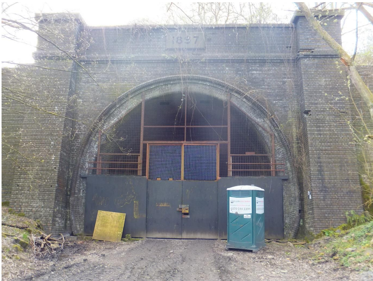
Figure 1 Northern portal of the Catesby Tunnel (SP 5245 5960).
