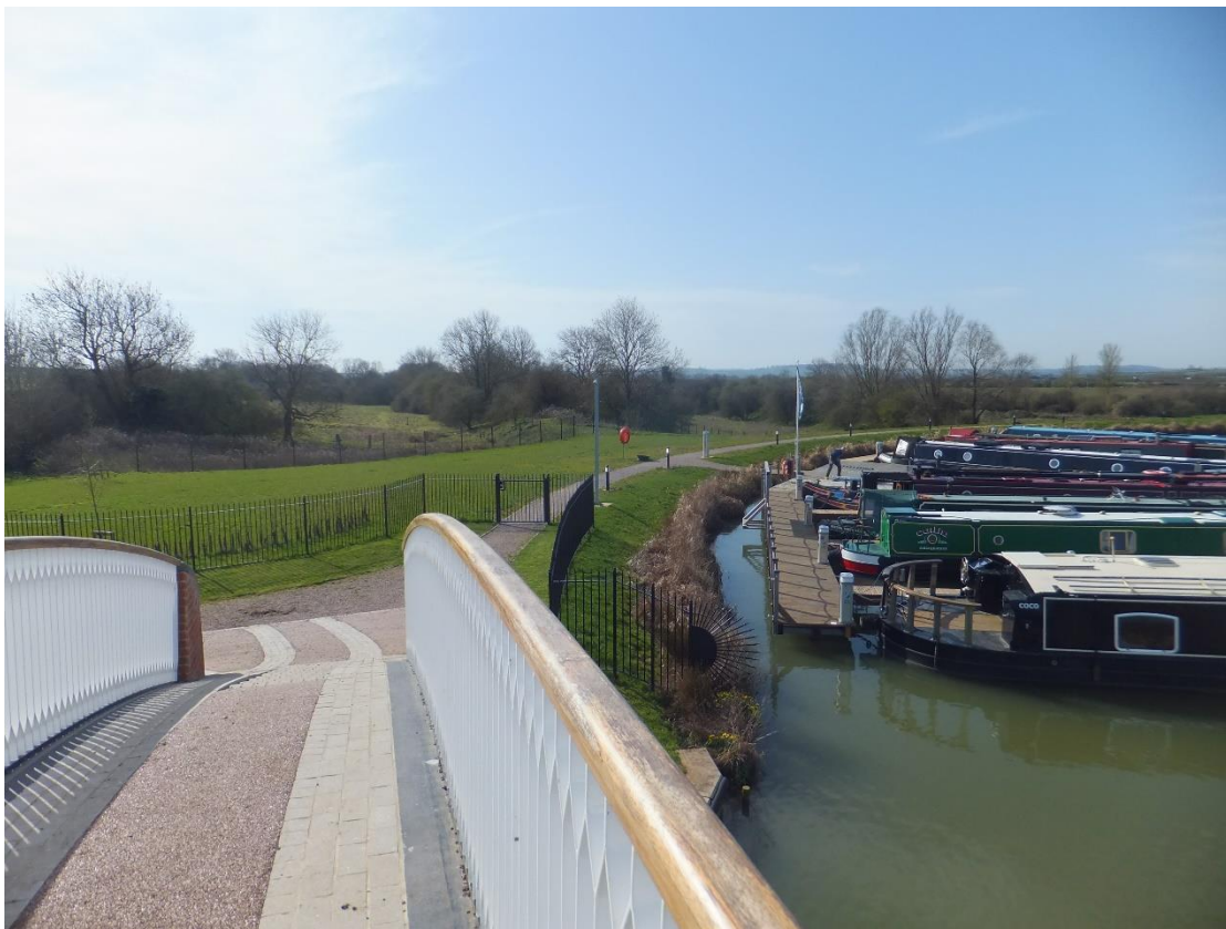
Figure 11 Looking south from the towpath bridge across the entrance to Dunchurch Pools marina. The northern end of the GCR embankment is visible ahead (roughly where the orange lifebelt can be seen). (Camera at roughly SP 5202 6977).
