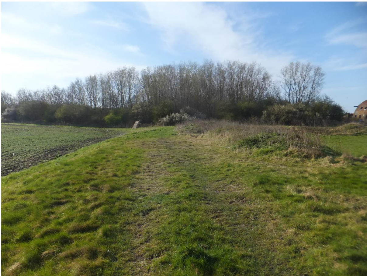
Figure 12 Looking south along the embankment of the GCR (SP 5185 7072).
