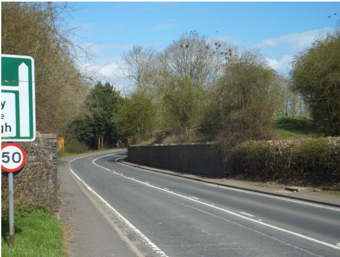
Figure 1 Looking north along the A45 east of Willoughby at the point where the GCR would have crossed on a bridge, with the embankment continuing northwards behind the wall (missing bridge at SP 5240 6718).
