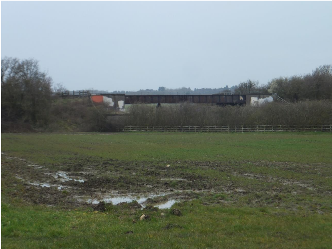
Figure 16 Looking west at the GCR bridge across the M45 (SP 5180 7127).
