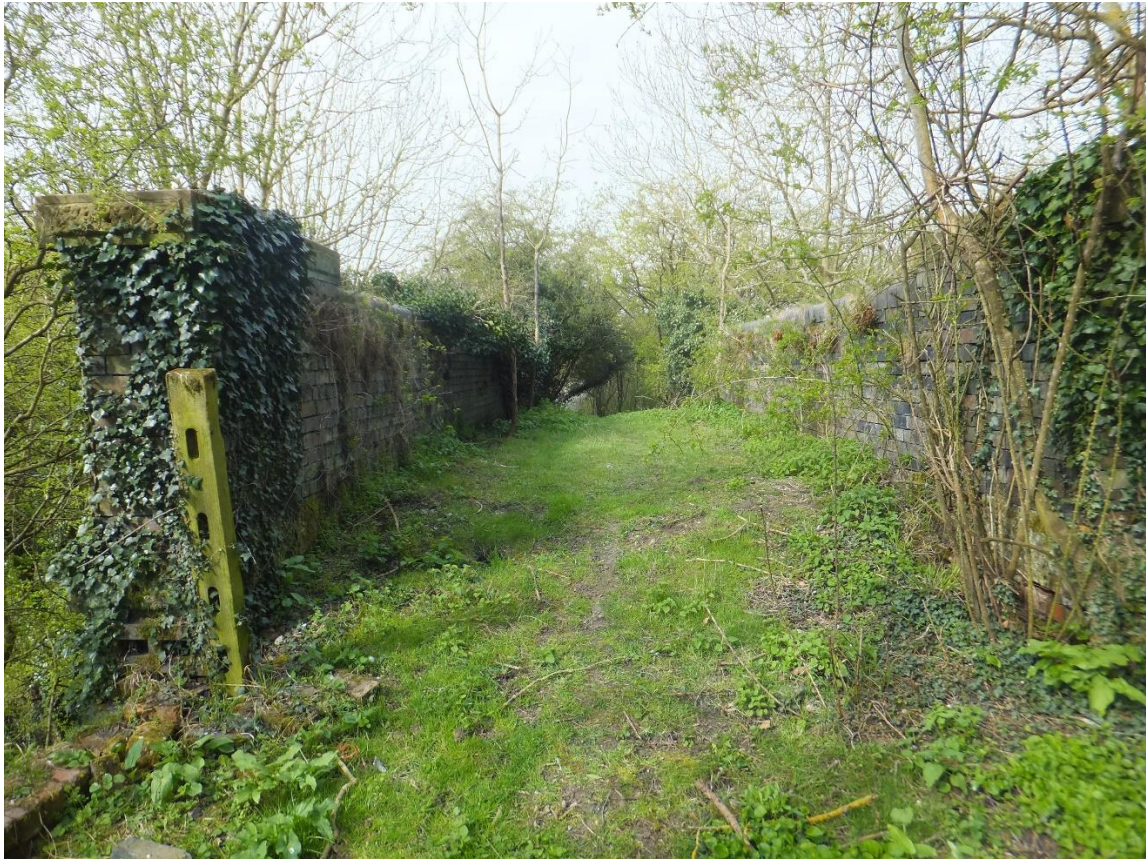
Figure 5 Looking west across the bridge over the GCR trackbed (SP 5218 6879).
