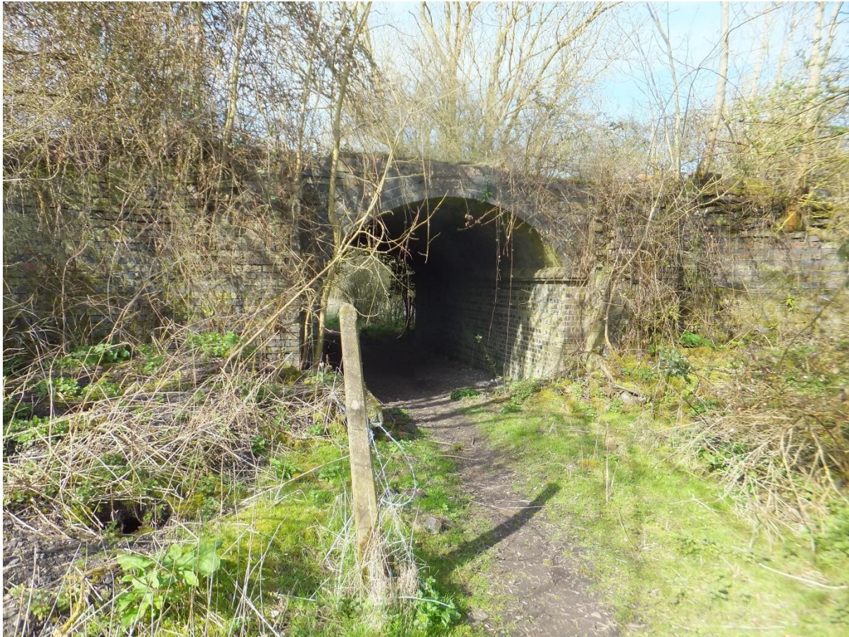
Figure 9 Looking west at a bridge carrying the GCR (SP 5204 6951).
