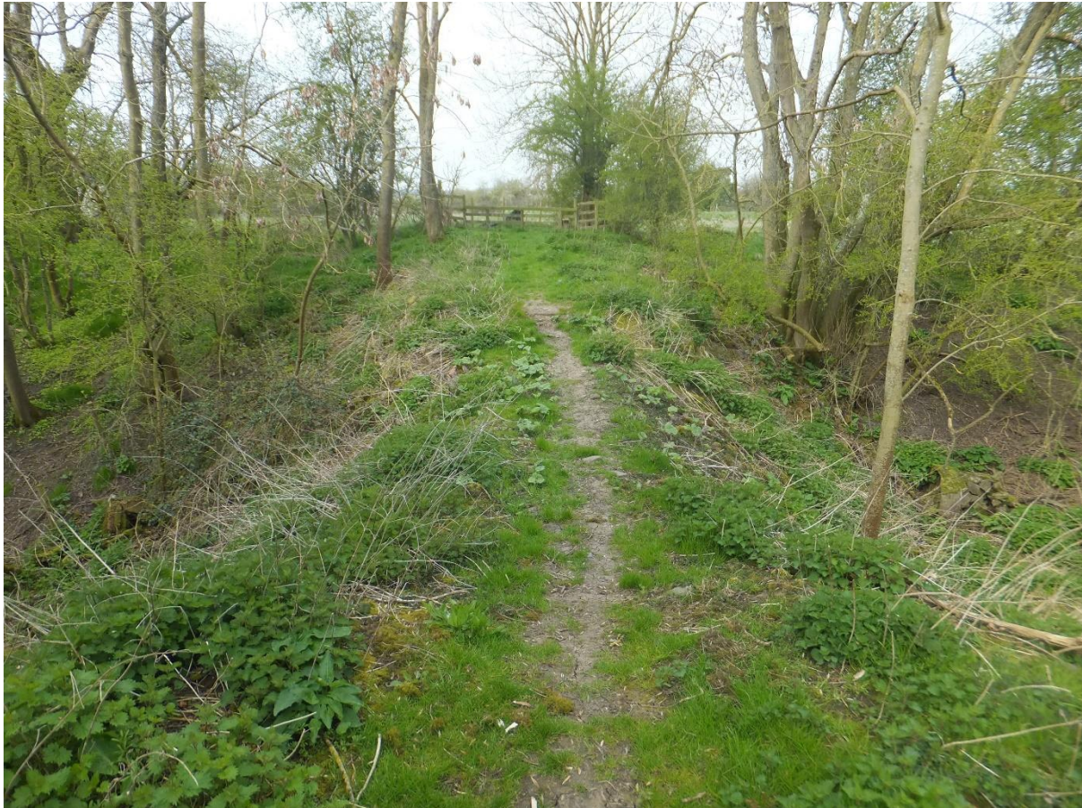
Figure 7 Looking west across the trackbed where the cutting is filled in, and a footpath crosses (SP 5213 6905).
