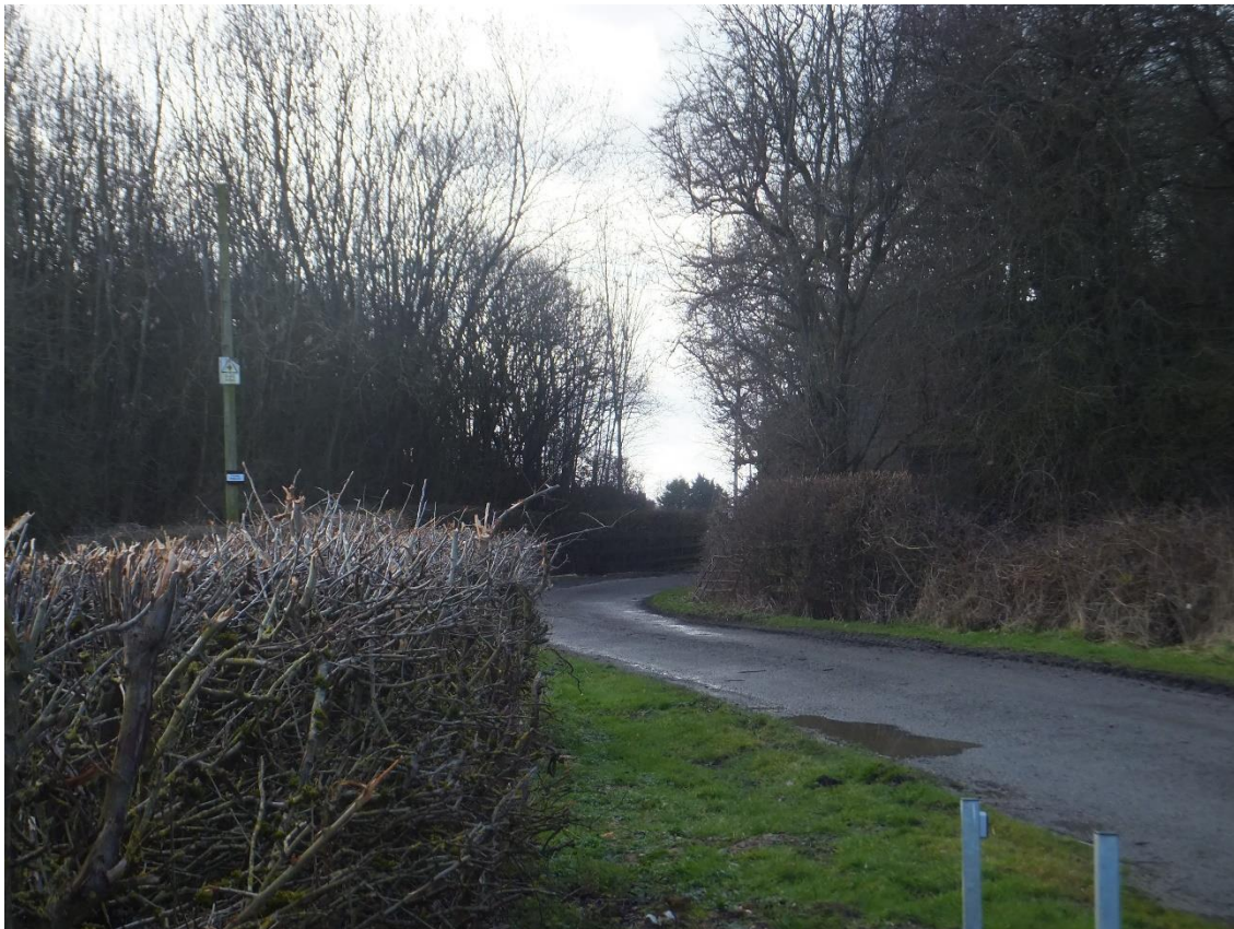
Figure 17 Looking west from the entrance to Lower Rainsbrook Farm at the point where a missing bridge would have connected the short embankment to the north with the longer embankment to the south (camera at SP 5172 7240).
